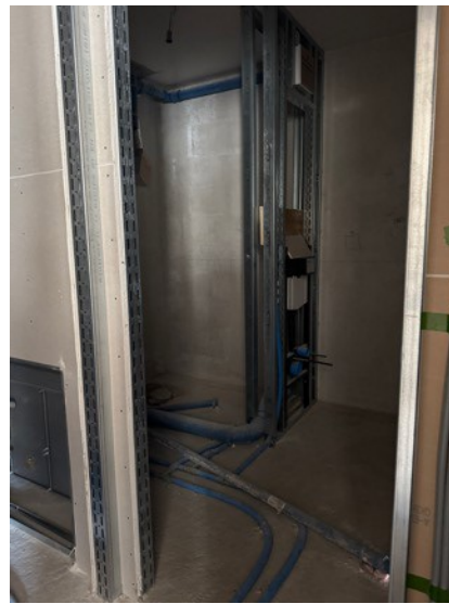
Erdgeschoss Top 2 – Bad (inkl. WC-Installation)
